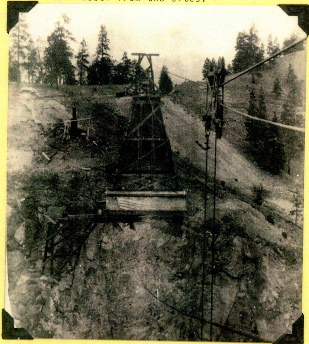
The first steps taken to build the Trout Creek Canyon Bridge in 1912. 985-2
