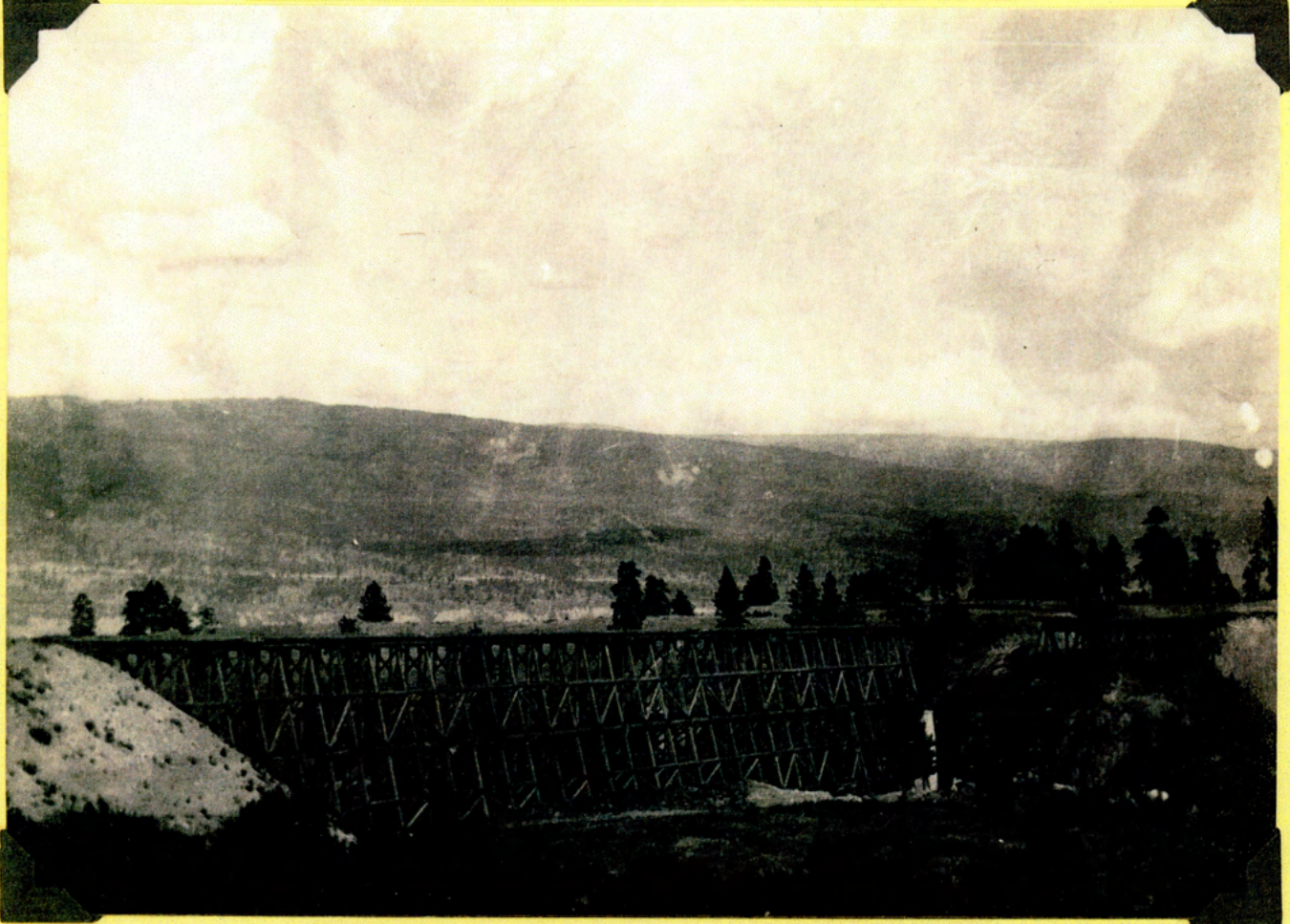
This picture shows the Trout Creek bridge nearly complete with track being partially laid. Picture taken circa 1914
